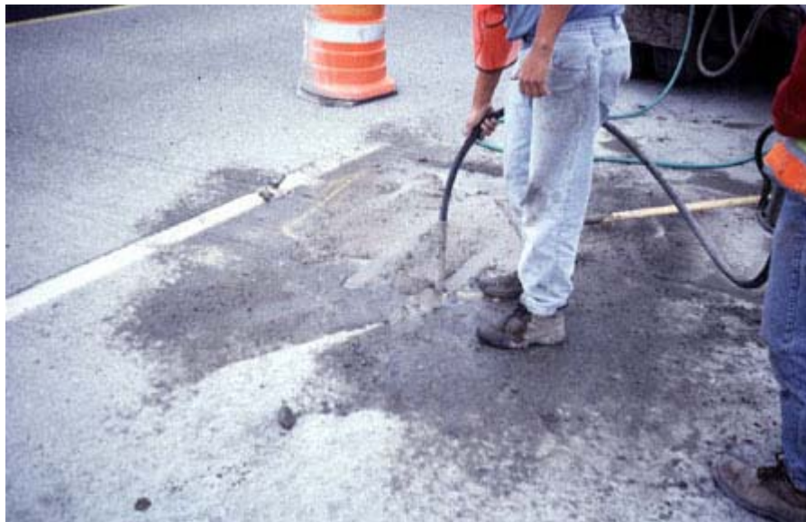
Figure 6-14 Consolidating backfill (Caltrans, 2006a)
