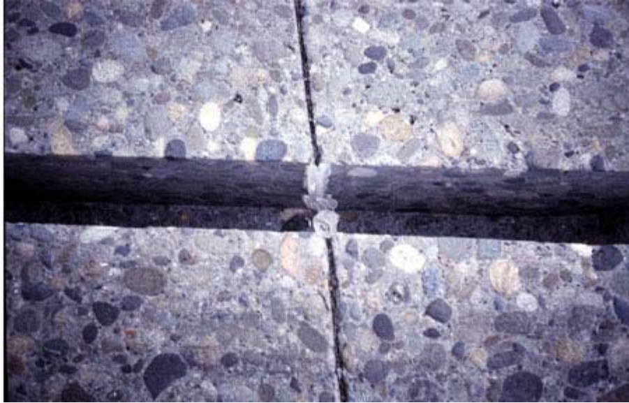
Figure 6-11 Sealing joint/crack (Caltrans, 2006a)
