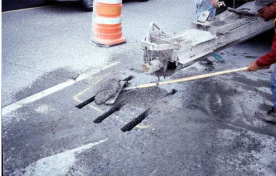
Figure 6-13 Placing backfill (Caltrans, 2006a)
