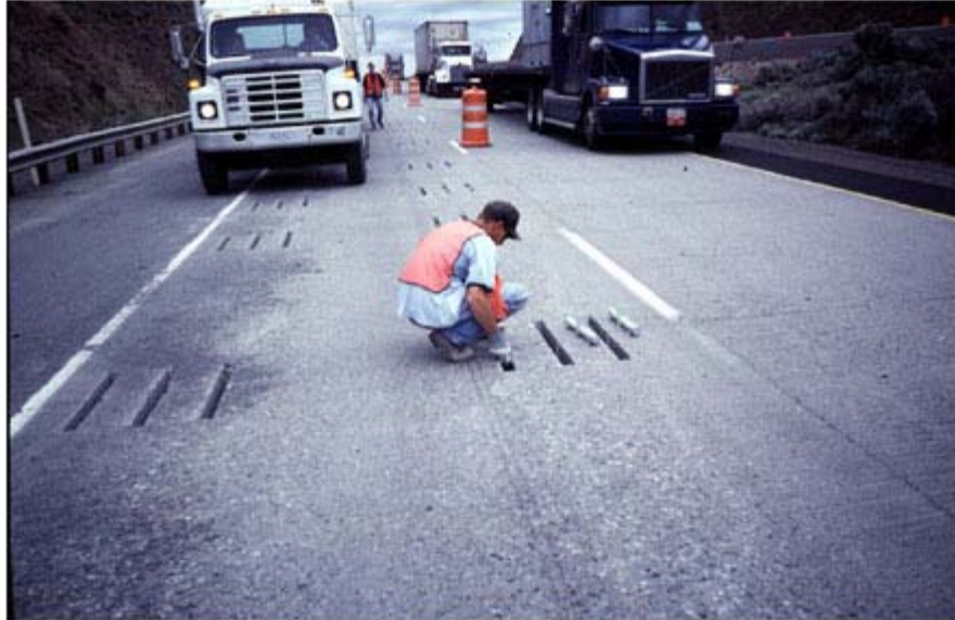
Figure 6-12 Placing dowel-chair assembly (Caltrans, 2006a)
