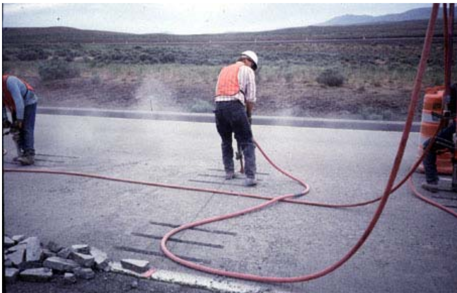
Figure 6-9 Jack hammering (Caltrans, 2006a)
